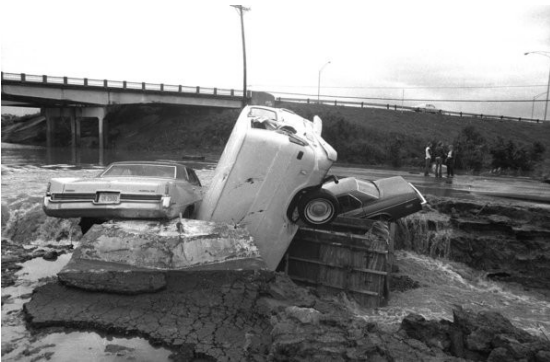
Damage from the 1974 Tulsa Flood (Photo Credit: Tulsa World)
