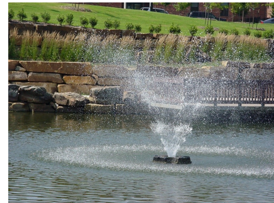
Aerating Fountain and Observation Dock (Outlet Structure)
