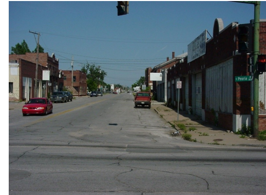
Existing Conditions on 6th Street
