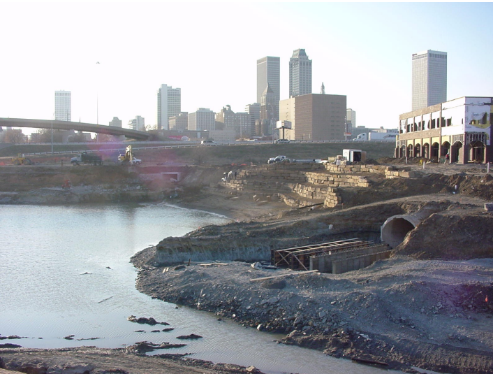
The new detention pond can be seen taking shape in this December 2005 photograph. On the right side of this view, the 108 inch diameter drainage pipe and new community center are visible.
