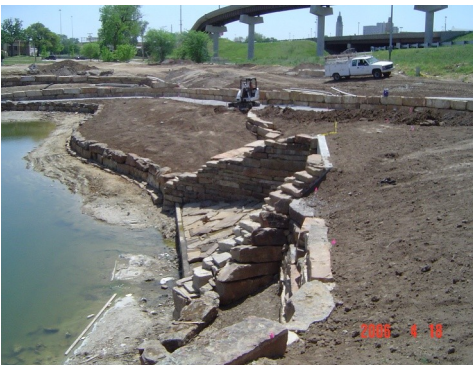
Natural stone was used to cover and visually disguise large concrete drainage structures.
