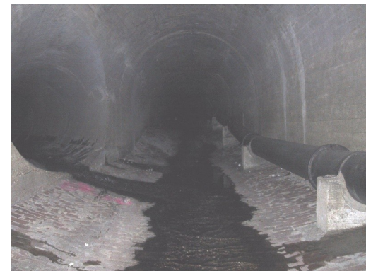
Elm Creek Arch Storm Sewer
