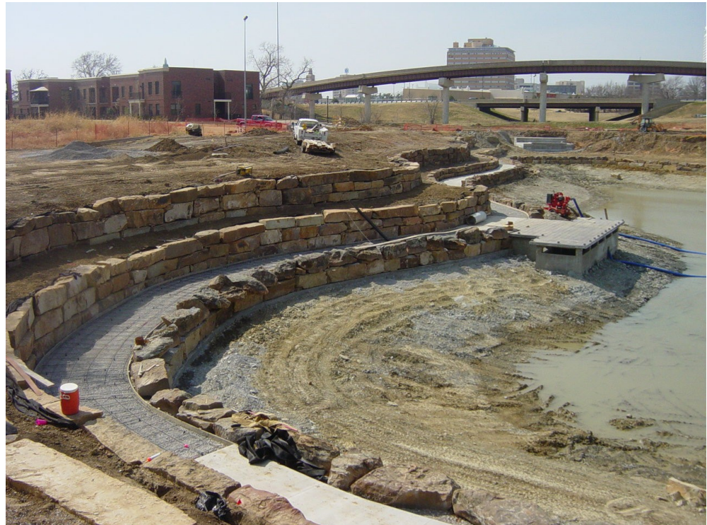
Large sandstone boulders were used to create a natural appearance where retaining walls were needed. Adjacent to the new pond, a boulder edge and lower level walkways were constructed to enhance views for park users.
