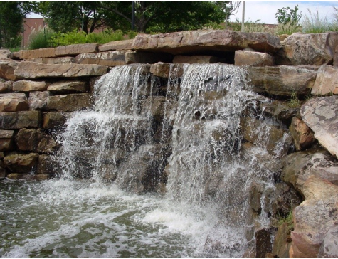
The stream begins with a 7 ft. tall waterfall which can be viewed from a large seating plaza. Lake water is pumped to this fall through two 7 hp submersible pumps.
