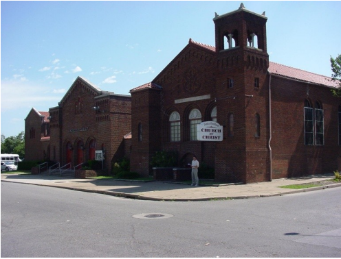
The Tenth and Rockford Church of Christ is an important neighborhood institution that abuts the west edge of proposed stormwater improvements.
