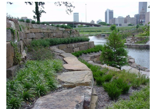
Sandstone boulder walls were terraced for safety and to create opportunities for landscaping.
