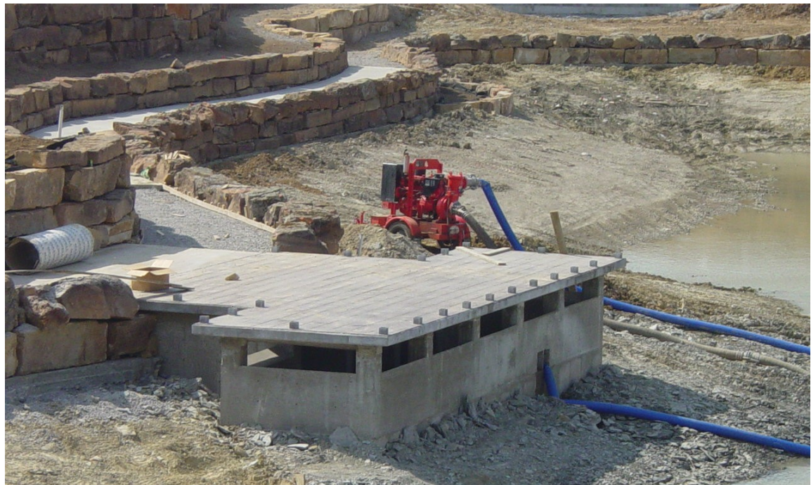
The primary outlet structure was nearly complete by March 2006. The horizontal edge of the weir opening maintains a constant water surface elevation in the pond and the cantilevered dock further contributes to the illusion of a dock constructed over piers into the water.
