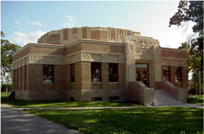
Figure 25: Tulsa Fire Alarm Building. Photo: David Stapleton
