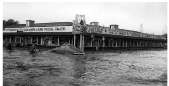
Figure 10: Storm water flooding the intersection by Hanna Hardware & Lumber on the southwest corner of 3rd & Peoria, circa 1952. Photo: Beryl Ford Collection
