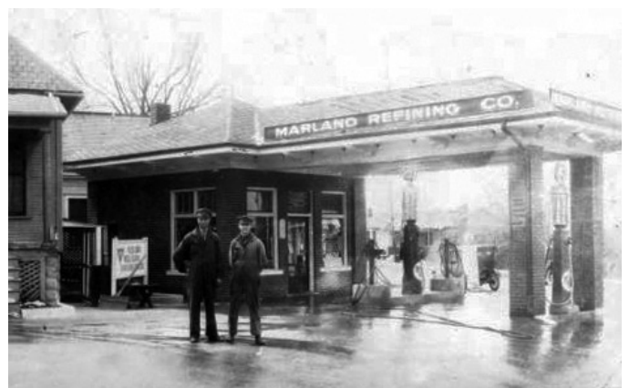
Figure 20: The Marland filling station at the northeast corner of 6th & Peoria. Photo: Beryl Ford Collection
