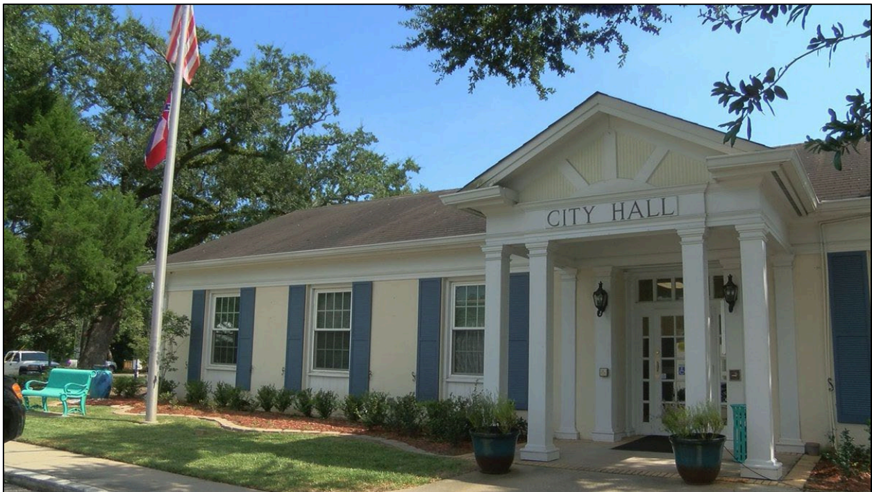
(Ocean Springs City Hall, located on the sole parcel in Area 6)
