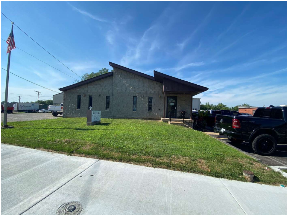
Brentwood Public Works Building, Ex.28 at P_00916.
