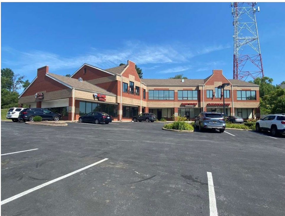
Office building, id. at P_00982.
